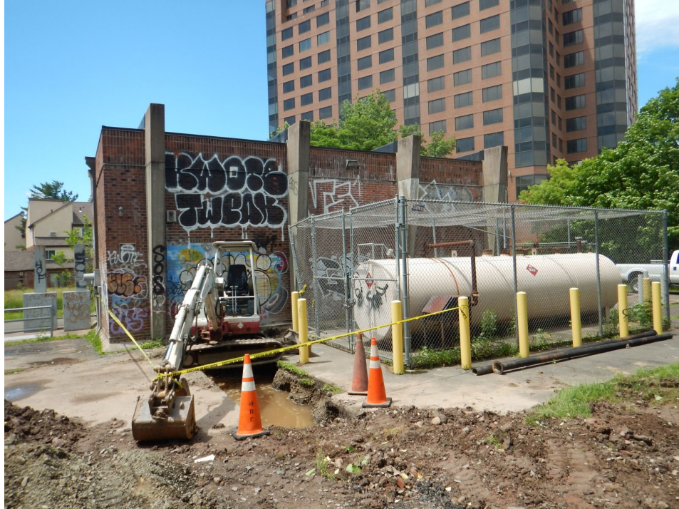
Figure 42: The Pope Pump Station and Fuel Tank; Maintenance Work in Progress
