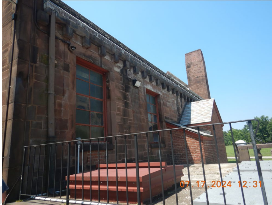
Figure 45: The Bushnell Pump Station
