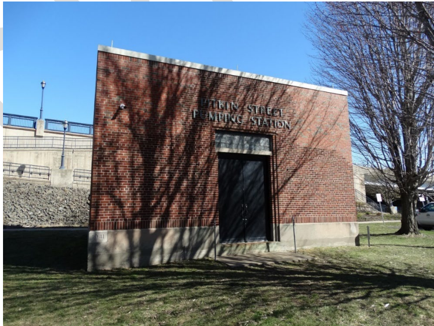
Figure 58: The Pitkin Street Pump Station
