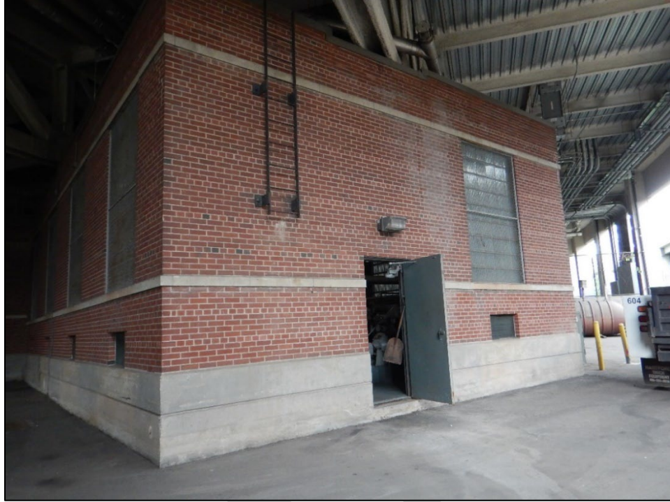
Figure 47: The Keney Lane Pump Station (Reserve Fuel Tank Outside the Main Building)
