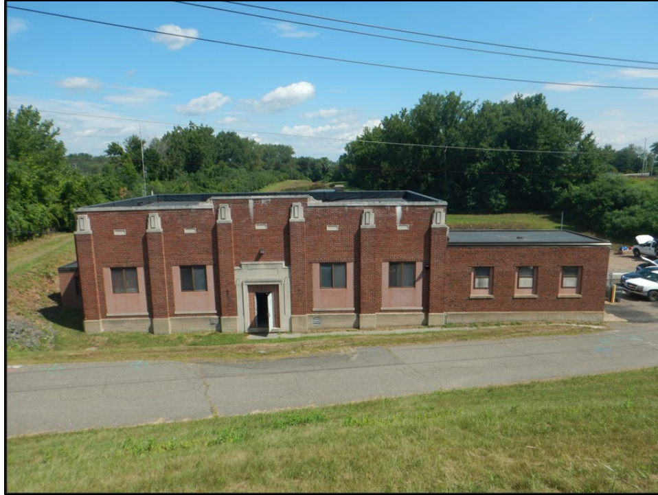
Figure 49: The South Meadows Pump Station
