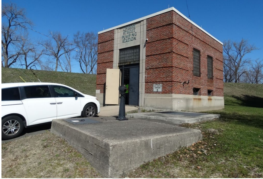
Figure 57: The Cherry Street Pump Station.
