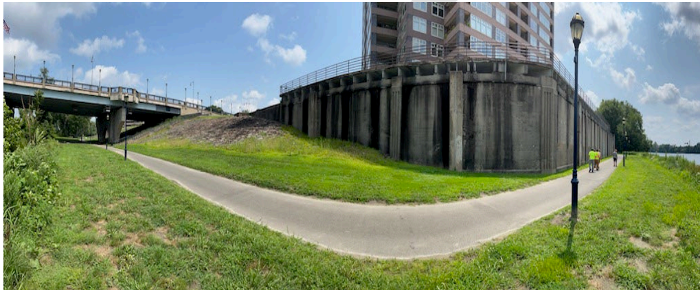
Figure 60: Riverpoint Condominium Complex Rising Above the Floodwall
