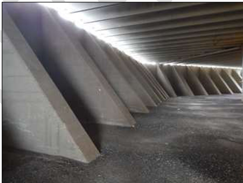
Figure 61: A Landside View of the Floodwall at the Riverpoint Condominium Tower
