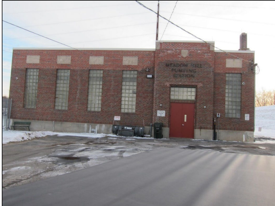
Figure 38: The Meadow Hill Pump Station
