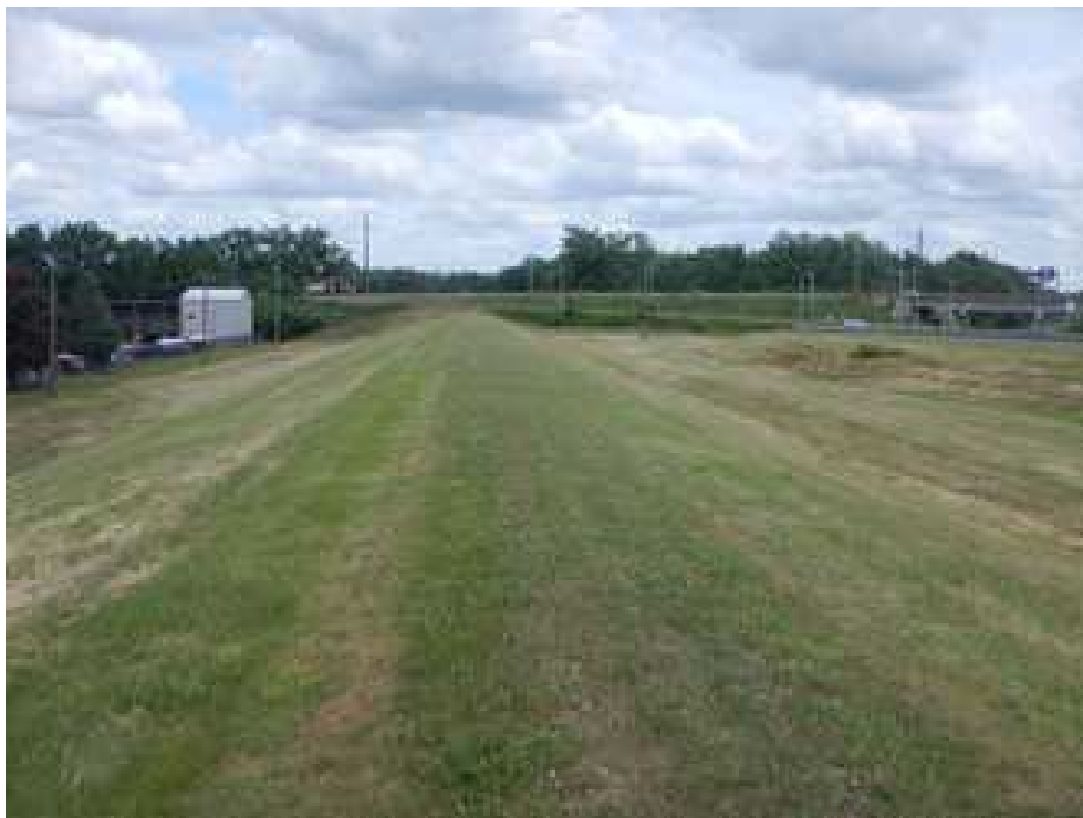
Figure 62: The Condition of the Levee Adjacent to Connecticut Natural Gas Corporation
