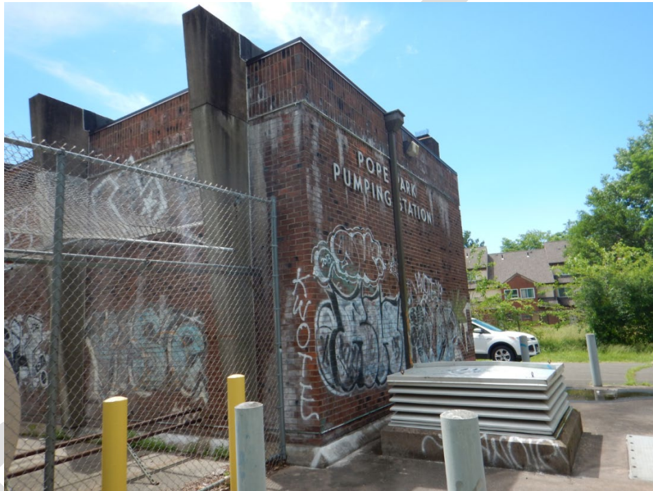
Figure 41: The Pope Pump Station
