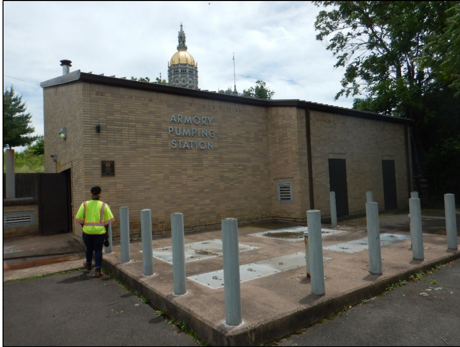
Figure 43: Armory Pump Station
