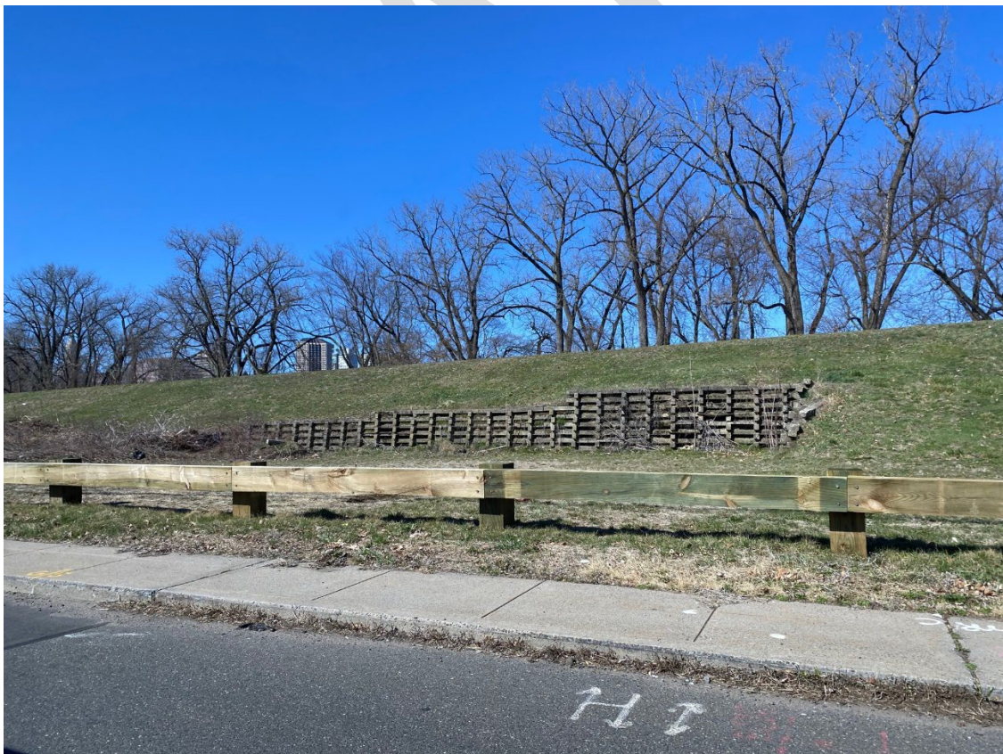
Figure 59: The Crib Wall in Segment 2 of the East Hartford Levee System
