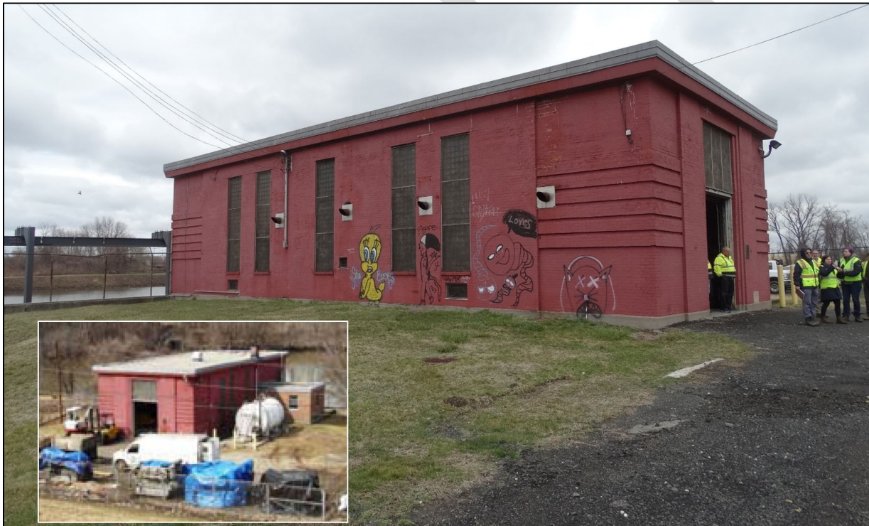
Figure 40: North Meadows Pump Station ( Inset, from 2009 inspection, shows the fuel tank and the shed housing the emergency generator )
