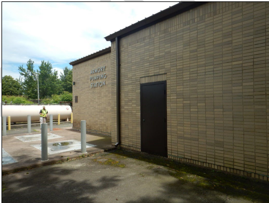
Figure 44: Armory Pump Station and Reserve Fuel Tank
