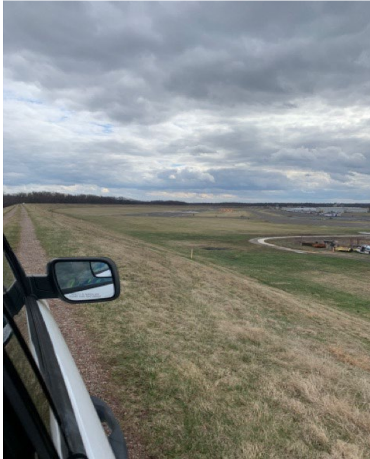
Figure 35: Levee Embankment Near the Hartford-Brainard Airport
